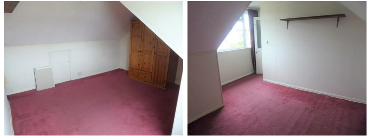
Rear aspect double glazed window, eaves storage space.
